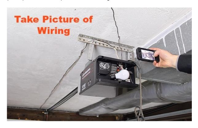
This gives you a reference for the new opener's wiring setup.
